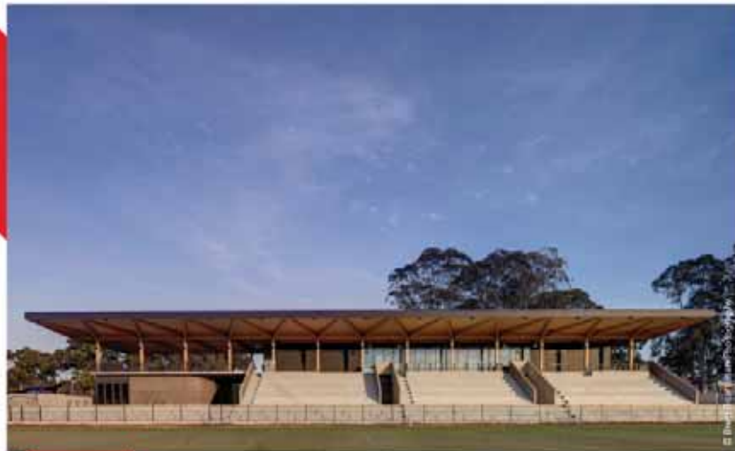
Eric Tweeddale Stadium, Cumberland, Sydney - the first project in Australia, where glued laminated timber is being used for the construction of a sports stadium instead of steel and concrete.
