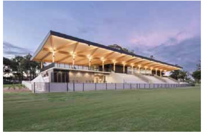
The Eric Tweedale Stadium in Western Sydney (above and below).
